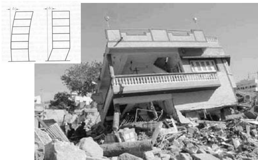
Figure 3.7a – Typical soft storey and torsion collapse in Bhuj
