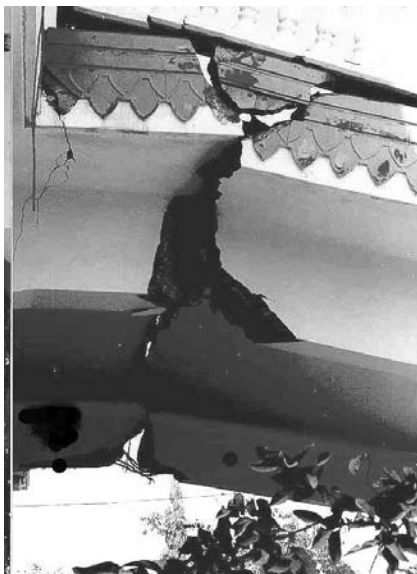
Beam Fracture
