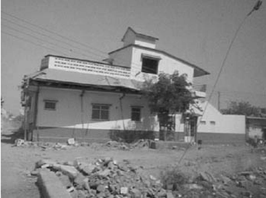
Figure 3.8 – Soft storey second floor collapse in Sukhpur
