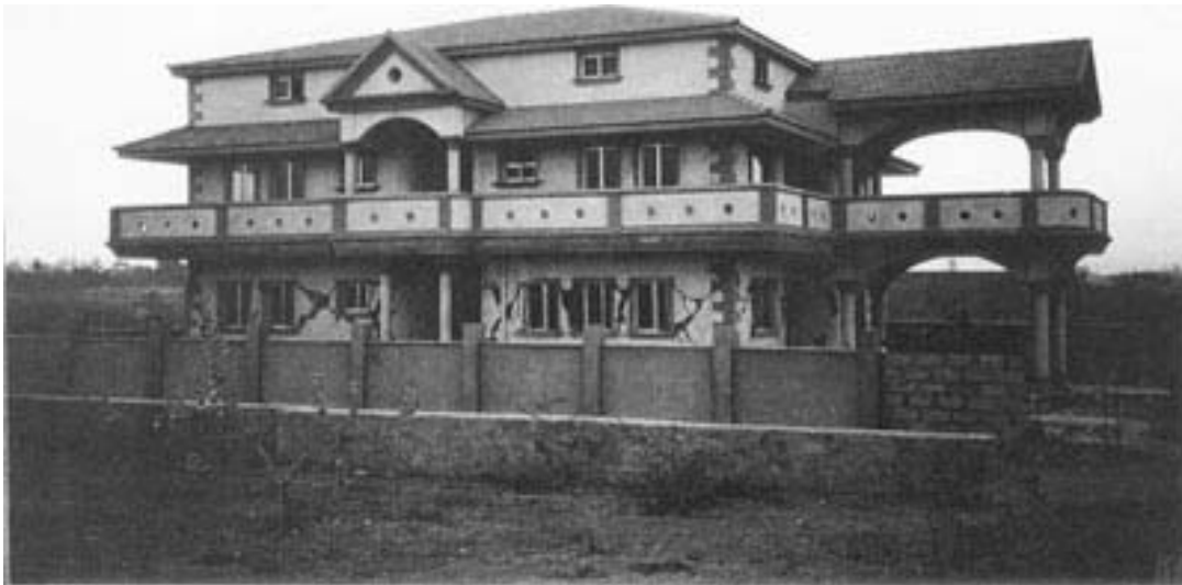
Figure 3.19 Damage to completed building after earthquake
