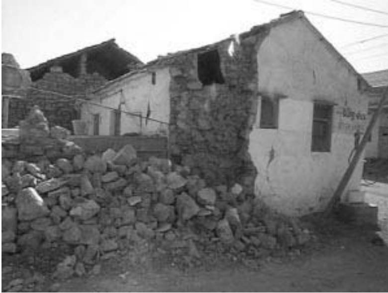
Figure 3.2 – Partial collapse of gable wall for a single storey random masonry wall in Kera
