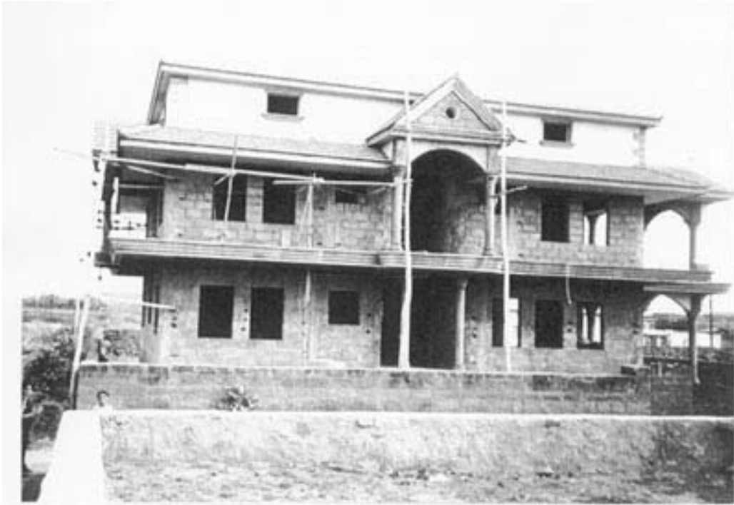
Figure 3.18 Building under construction one year prior to earthquake
