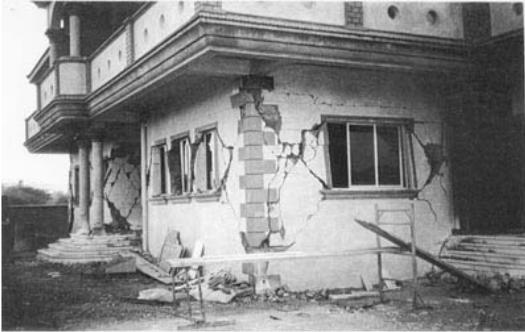
Figure 3.20 Large window openings close to corners and short column failures
