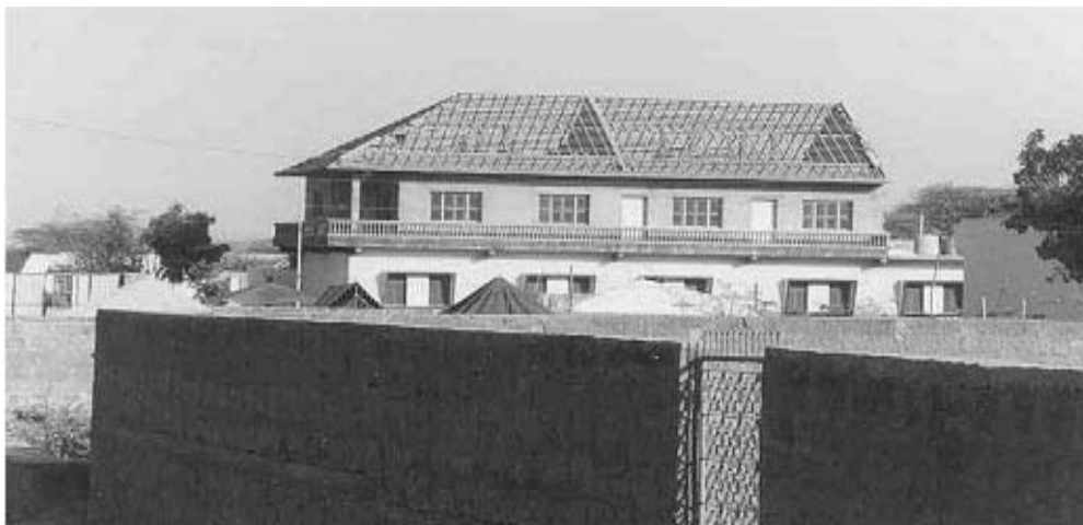
Figure 3.10 Infill panels again prevented collapse of this structure although all the roof tiles fell off - Mirzapur.
