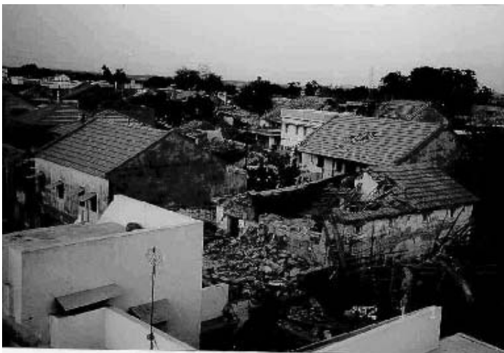
Figure 3.1- Collapse of random masonry building in Manukawa
