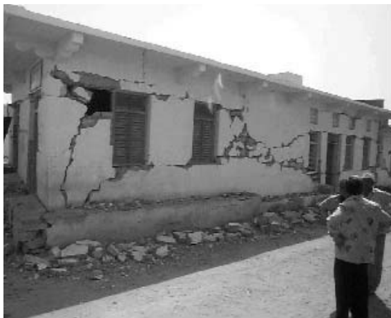
Figure 3.2 – Partial collapse of gable wall for a single storey random masonry wall in Kera
