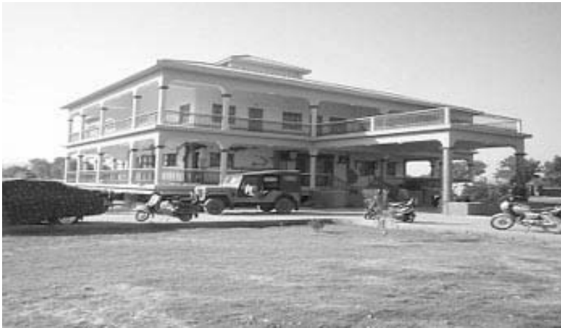
Figure 3.9 Infill panels to an reinforced concrete frame building acting as non-structural shear walls, provided stability to the overall frame – Bharasar
